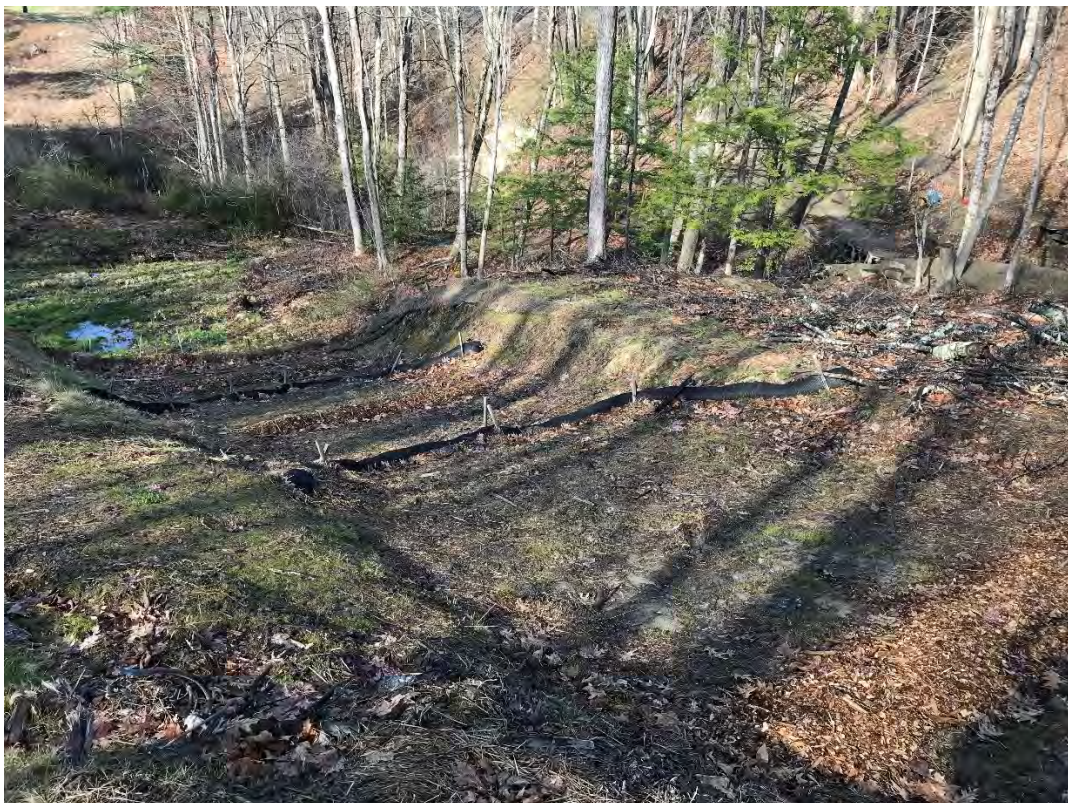
Fig 8: Lower portion of slope between Strs. 28 and 29. Viewing northeast. (04-19-21)
