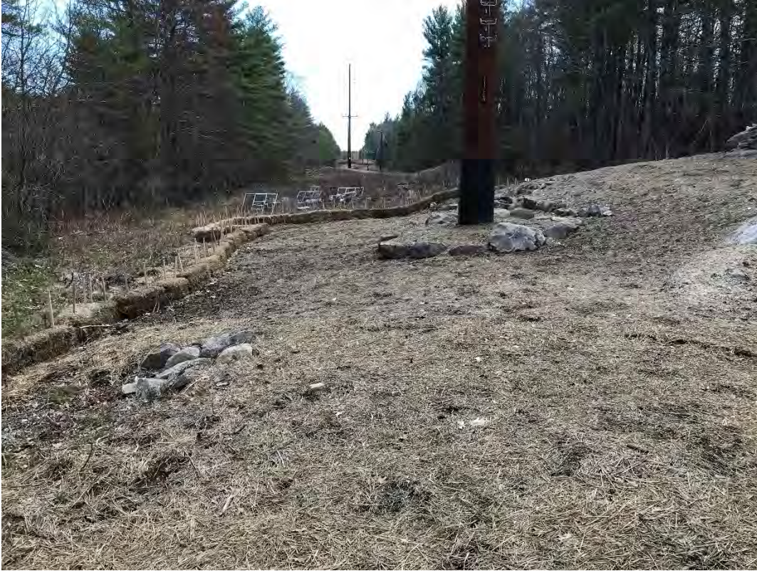
Fig 5: Str. 89 work area. Viewing southeast. (04-19-21)
