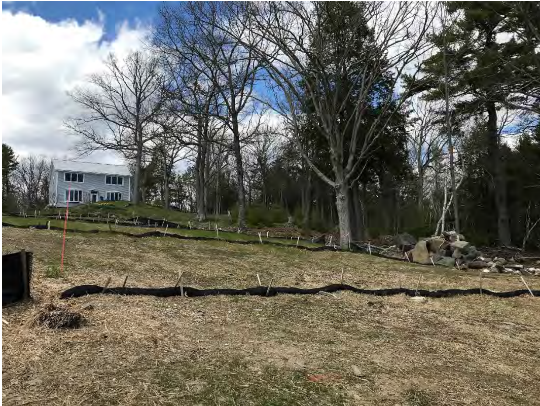
Fig 3: Slope above the cable house at the west side of the bay. Viewing northwest. (04-19-21)
