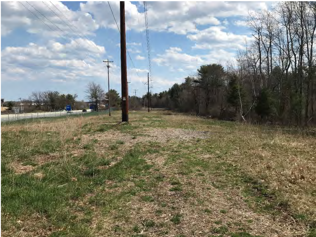
Fig 18: Str. 123 work area. Viewing southeast. (04-20-21)
