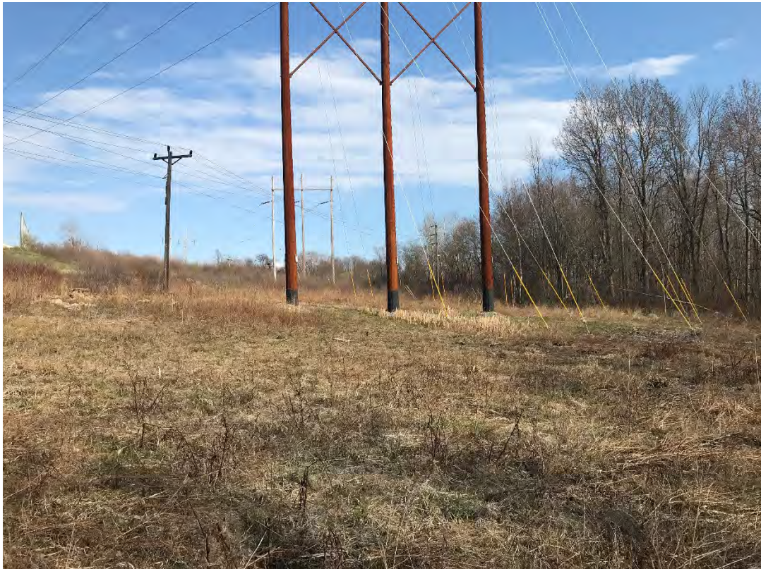
Fig 14: Str. 143 work area. Viewing east. (04-20-21)
