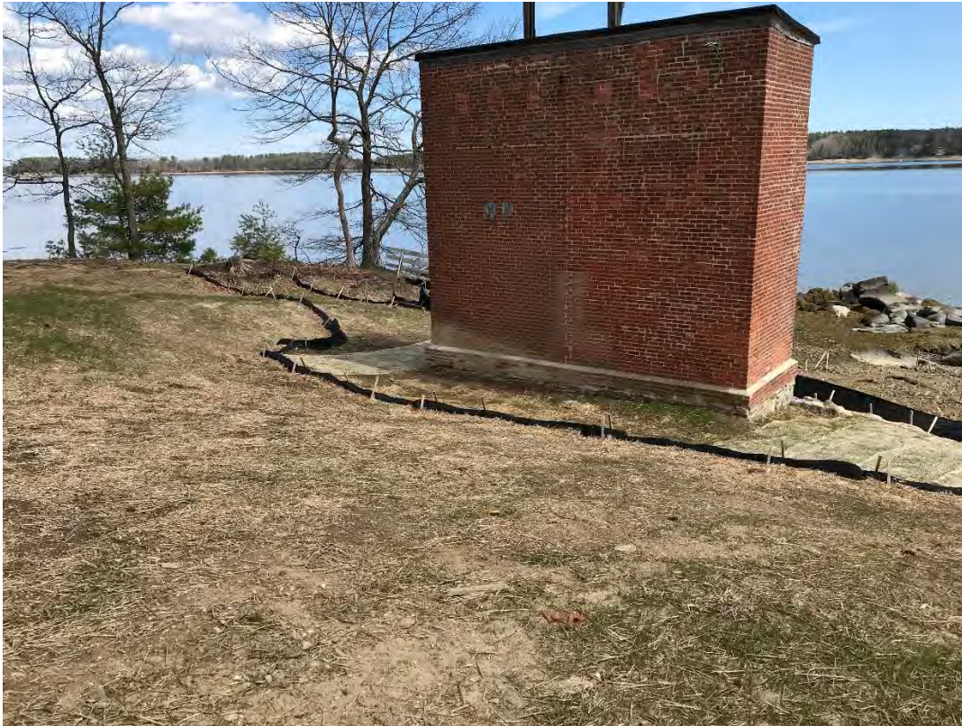
Fig 1: Slope leading down to cable house and salt marsh restoration at the west side of the bay. Viewing northeast. (04-19-21)
