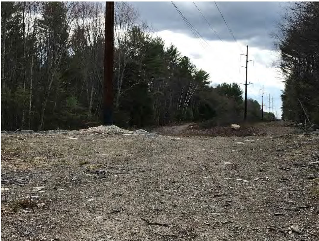
Fig 16: Str. 78 work area. Viewing southwest. (04-19-21)
