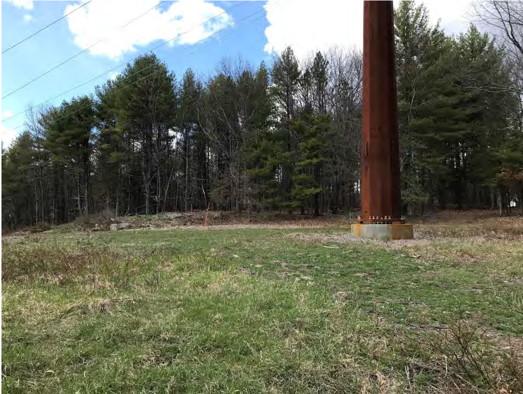
Fig 15: Str. 85 work area. Viewing northwest. (04-19-21)
